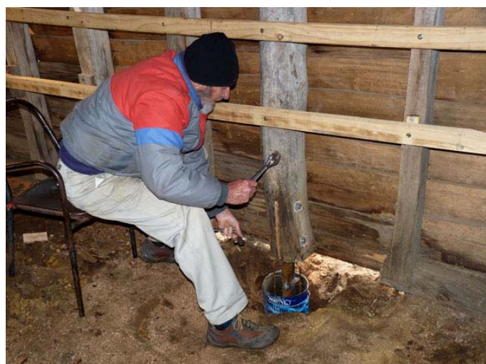
Photo: No OH&S concerns here - Pat restumps in comfort.
