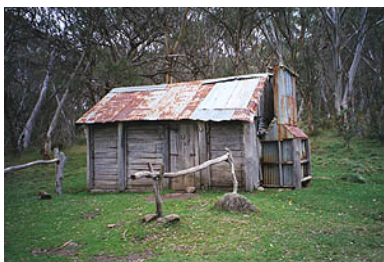
Photo: Cascades Hut, built in 1935 originally with bark roofing and regularly restored and maintained by IAC with permission from NPWS
